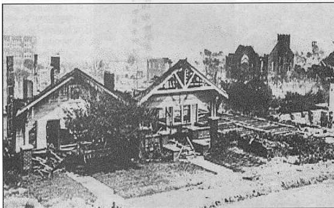
These burnt out houses nevertheless give an idea of what many homes in Greenwood looked like. Manicured lawns, lovely brick and framed houses.
