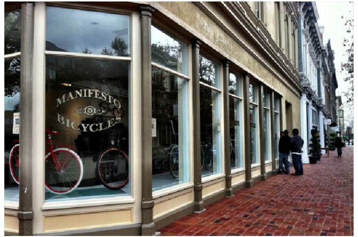
Manifesto Bicycles is one of six stores in Oakland's Popuphood. Credit: Oakland North
