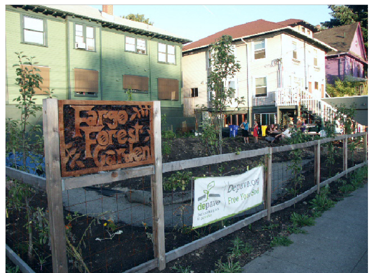
The Fargo Forest Garden replaced 3,000 square feet of asphalt. Credit: Picasa user DepavePDX
