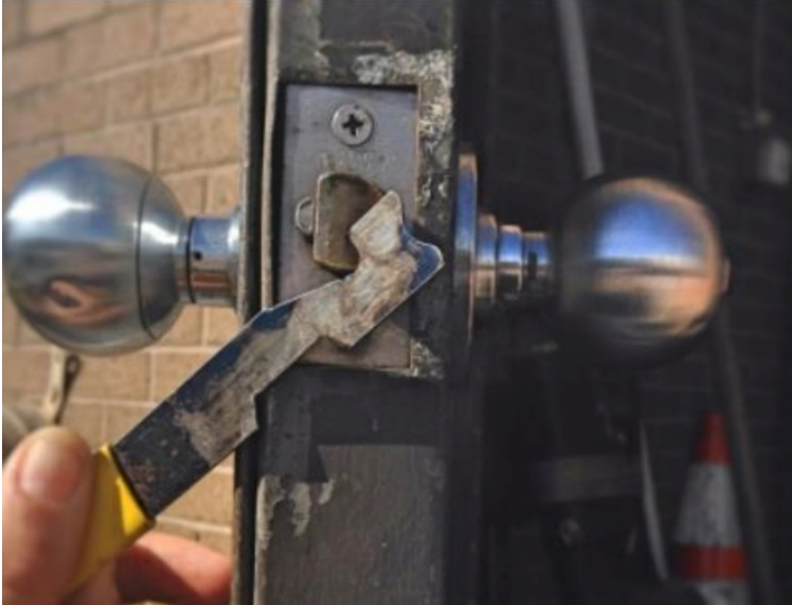
How a Shove-it Tool Bypasses a Latch
