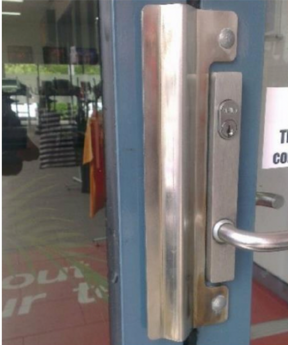
Large Strike Plate Cover Over Large Door Gap
