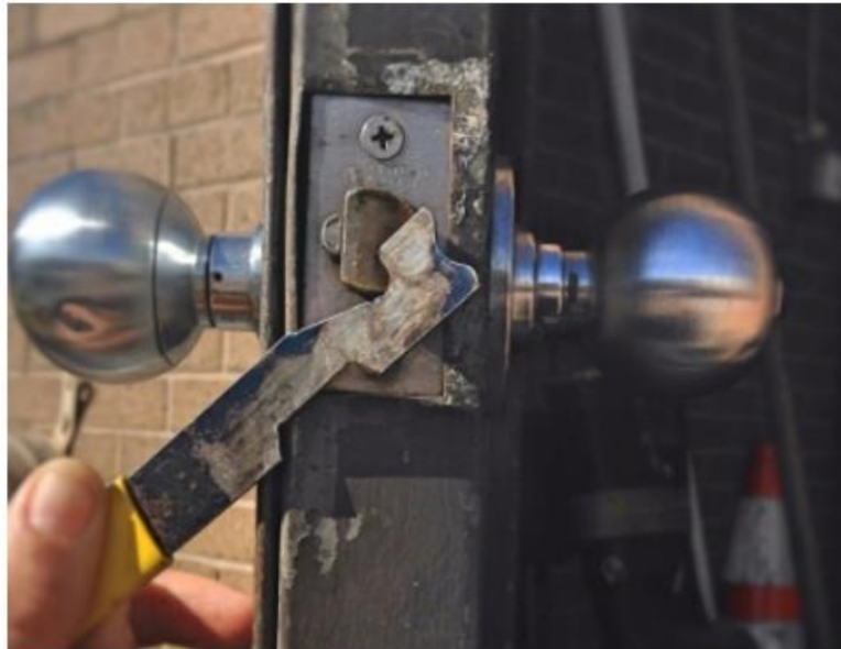
Figure 72. How a Shove-it Tool Bypasses a Latch
